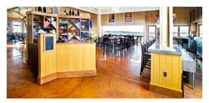
The two main bars in the restaurant were cast-in-place. The main bar is straight and is 32' x 2'6" and the curved kitchen bar is 35' long by 3' wide and has a light dosing of blue and green glass exposed in the surface. We custom batched our materials on site and finished the surface with a hard trowelled surface.
