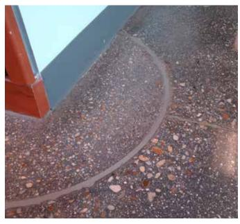
We processed over 8,000 sqft of polished concrete on an integrally colored slab. We worked very closely with the concrete subcontractor from pre-placement planning through final finish of the slab. This slab was challenging because the concrete used was a dark, integrally colored slab that would show every imperfection in the finished surface. To combat this, we made sure to fully refine the concrete with each pass to eliminate any inconsistencies in the surface.
